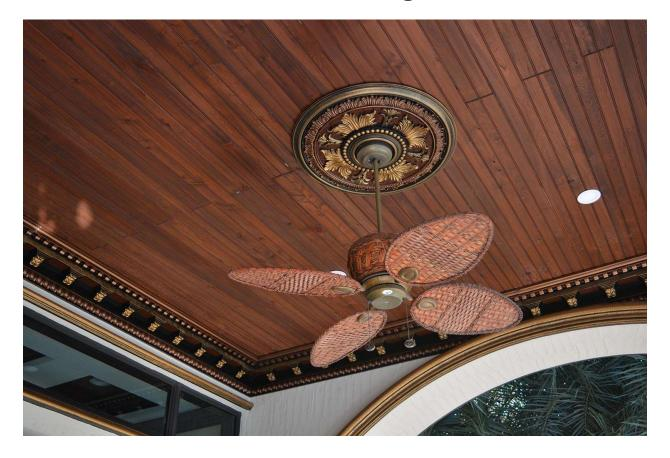
**Important:** If your Ceiling Medallion comes with no hole from factory, it should be cut prior installation, just choose the appropriate diameter of the hole you need to cut according your electric box size and the canopy of your ceiling fan or light fixture, also check the medallion specifications (center hole diameter and maximum that a canopy can fit) provided in the product page tabs. You can use a regular hole saw tool available in any local store to cut the medallion.
